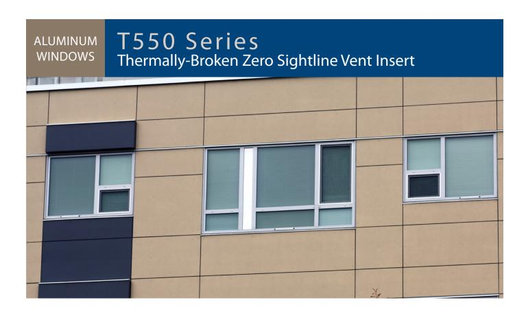
The D8 Aluminum T550 Series Thermally-Broken Zero Sightline Vent Insert is a glazed-in vent system that is available as both projected-out casement and awning configurations. The thermally-broken vent frames enhance thermal performance and incorporates glass that is structurally glazed to the operable sash which eliminates exterior sightlines.
